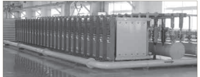
Example of a multi-bank installation
