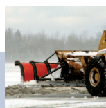
VVP Pressure valve on snow plow
