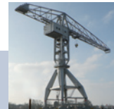
Harbour handling material
